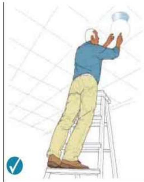
Correct – 3 clear rungs, do not work any higher on this type of stepladder
