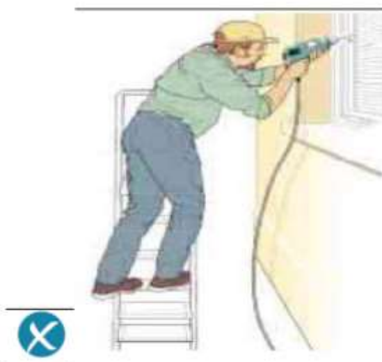
Incorrect – steps side on to work activity
